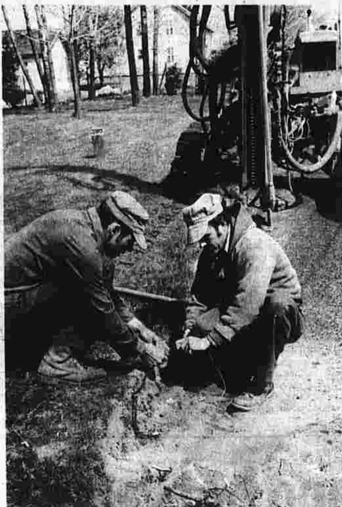
Keeney St. storm sewer work started
